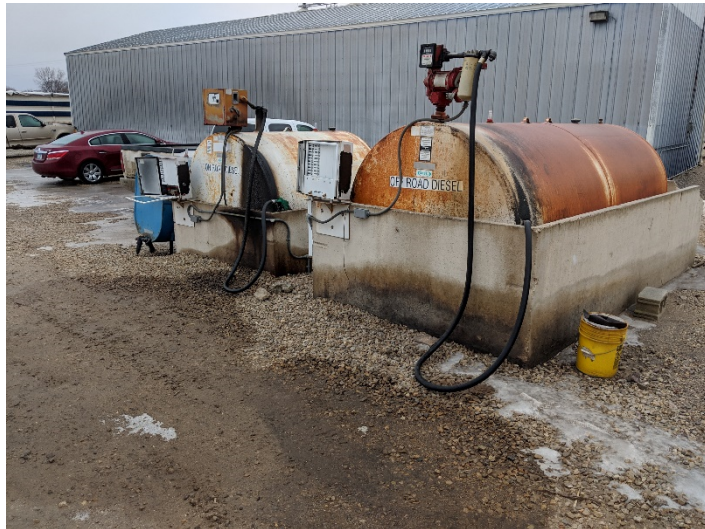
7) Diesel fuel ASTs and associated ground staining
