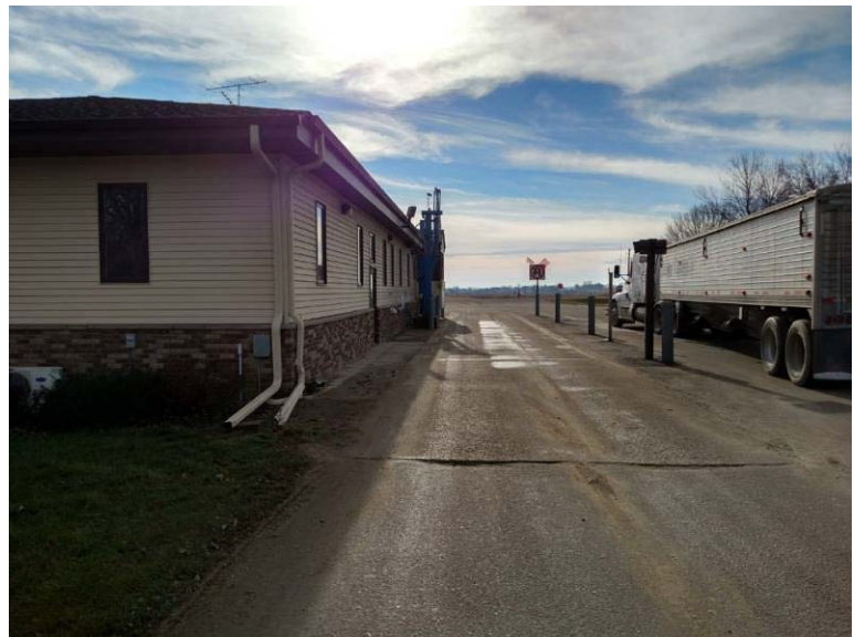
PHOTO 2. West side of office/scale house viewing south.
