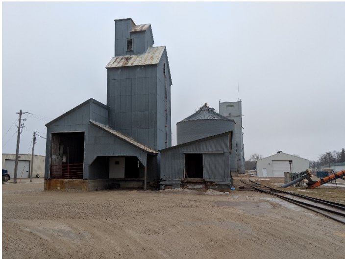
3) Historical grain elevator-no longer in use
