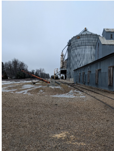
17) Rail spur along eastern portion of Subject Property
