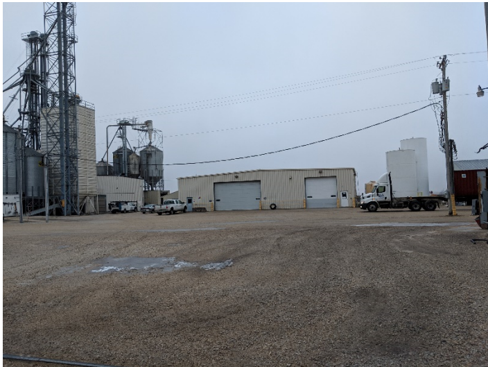
11) Maintenance shop and pole-mounted transformers
